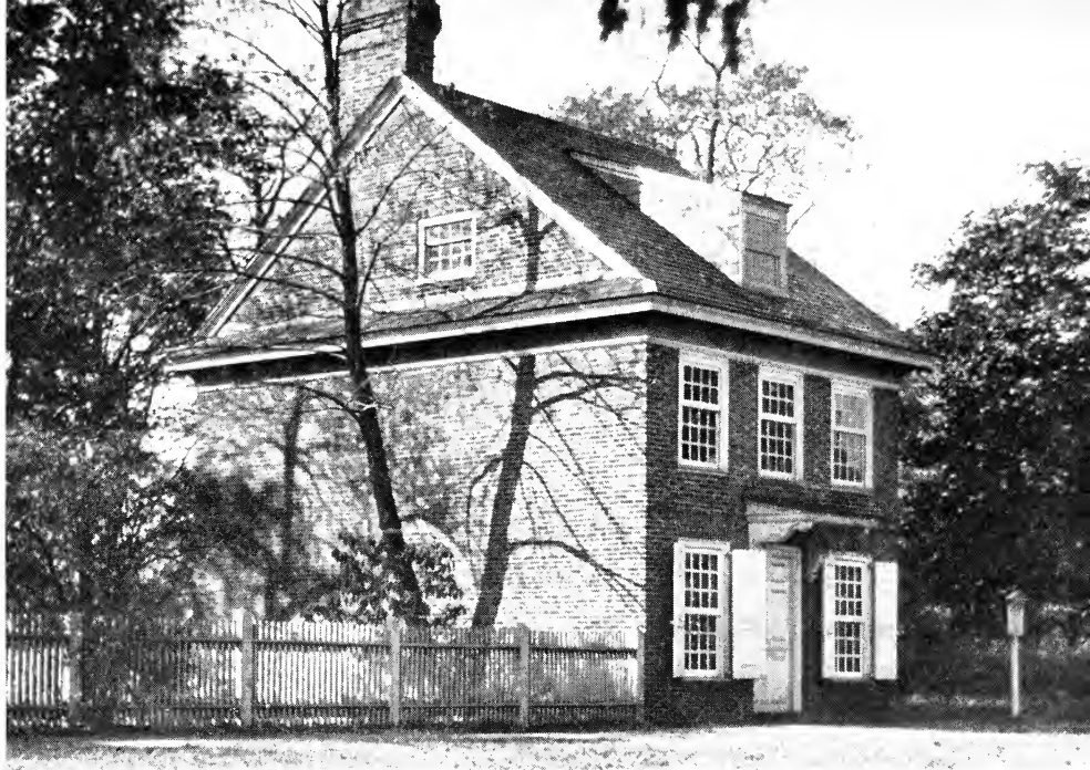
Exterior of Letitia St. House
